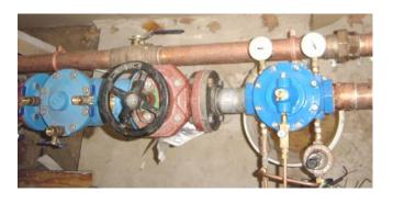
Typical installation of a Flomatic Model RPZ Backflow preventer on the main potable water line a head of a Model C101 (S/N 03634) Automatic Pressure Reducing Control Valve
