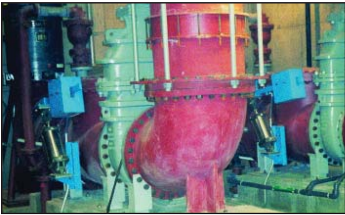
Boston Tunnel Project - "The Big Dig"
