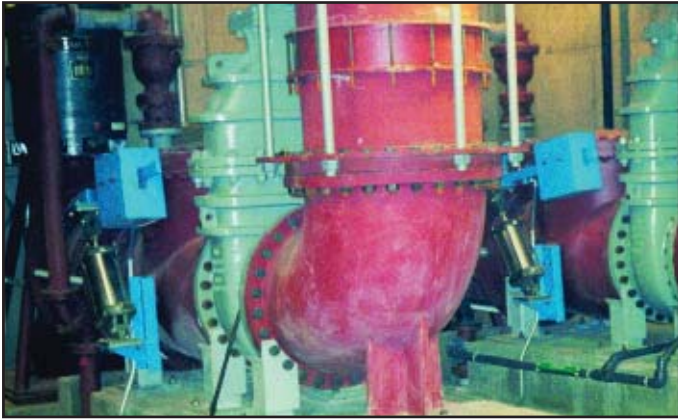
Boston Tunnel Project - "The Big Dig"
